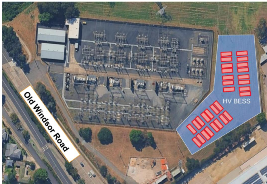
Figure 2: Aerial view of the Baulkham Hills substation and proposed HV BESS site
